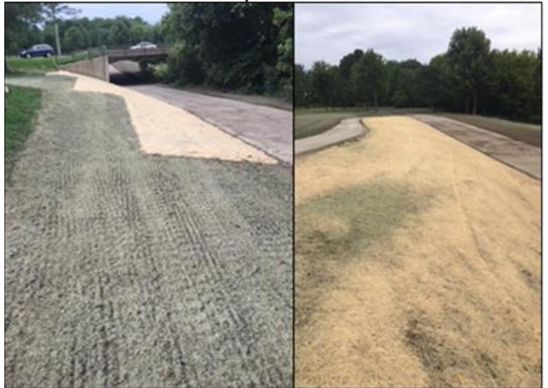
Drill lines in the left photo will provide good roughness to impede erosion while the proper hydromulch thickness was applied. The steeper slope to the right was covered with a woven blanket to provide good slope protection and integrity while vegetation works to take hold.
