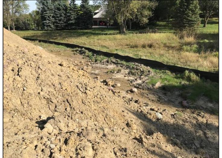
Silt fence and sediment traps in sequence were utilized at this site. One trap upstream of the pictured area helps lessen the load on the far trap and properly installed silt fence.
