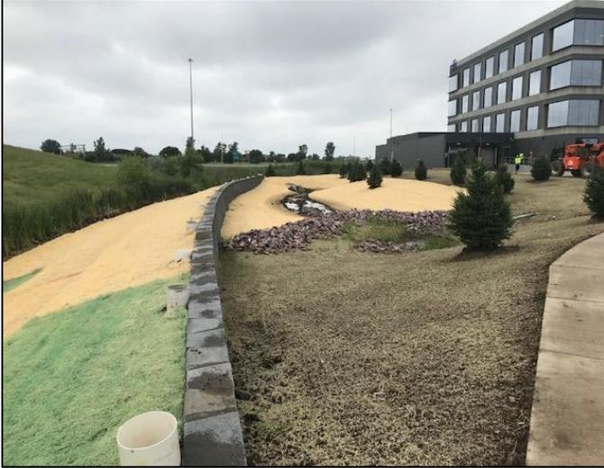
One of the three sediment basins at this site is pictured to show ideal stabilization of a basin and the slopes surrounding it. Proper hydromulch application and turf reinforcement has been utilized throughout.
