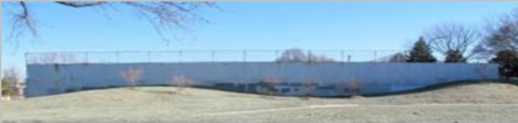
The existing wall in Meldrum Park
